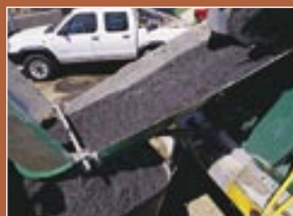
2 AFTER SUFFICIENT MIXING, COLOURED CONCRETE IS DISCHARGED FROM CONCRETE TRUCK
