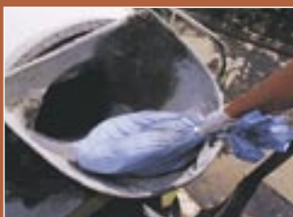
1 PREFORMULATED BAGS OF CCS PIGMENT CONCENTRATES ARE ADDED TO THE CONCRETE TRUCK AT THE PREDESIGNATED RATE OF ONE BAG PER CUBIC METRE
