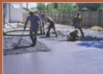
3 COLOURED CONCRETE IS SCREEDED AND FLOATED
